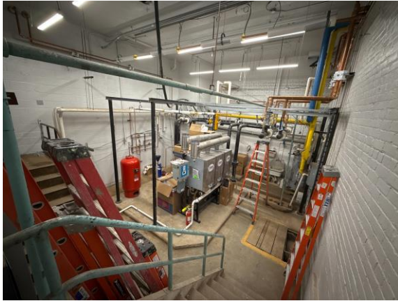
ECC – Boiler Room In Progress
