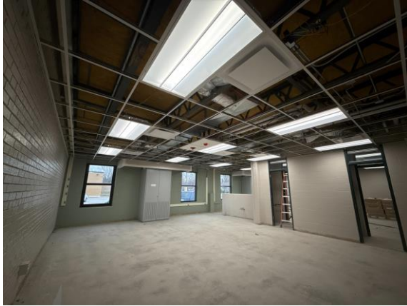
ECC – Classroom VUV Drywall Bulkheads In Progress
