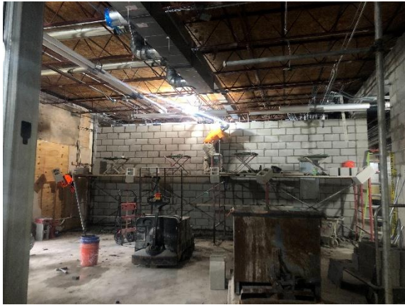
ECC – Future Main Office Masonry Wall In Progress
