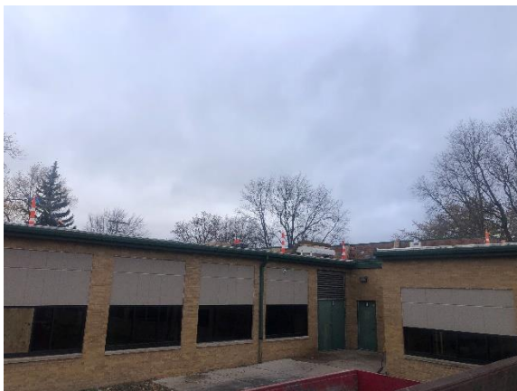
ECC – Big Chimney Demo Complete & Window Install In Progress
