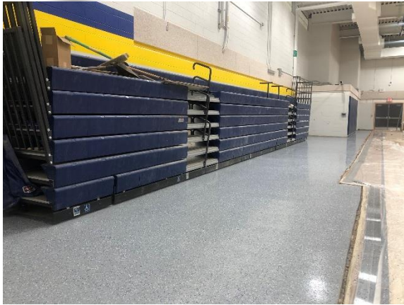
CES – Gym Addition Epoxy Floor Near Complete
