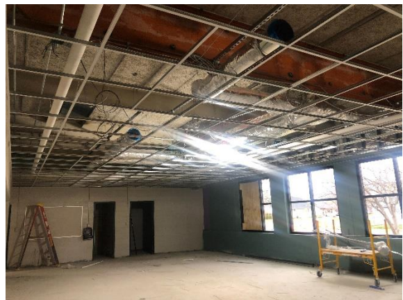
ECC – Area D Ceiling Grid In Progress
