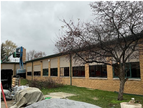
ECC – Big Chimney Demo & Window Install In Progress
