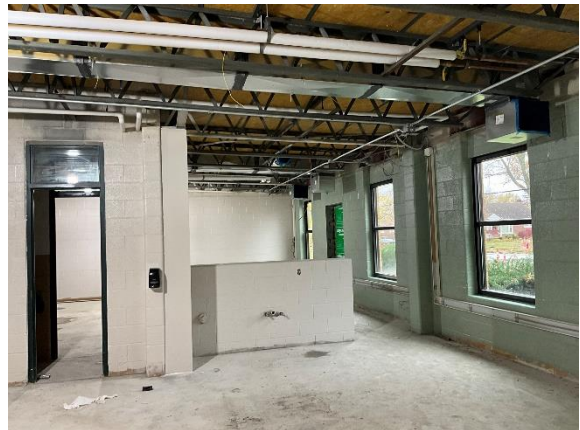
ECC – Area D Painting In Progress
