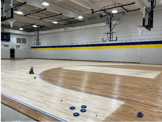
CES – Gym Addition Wood Finishing Near Complete
