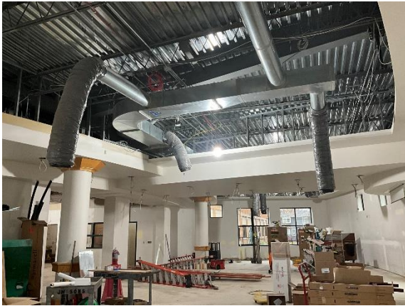
ECC – Library MEP In Progress
