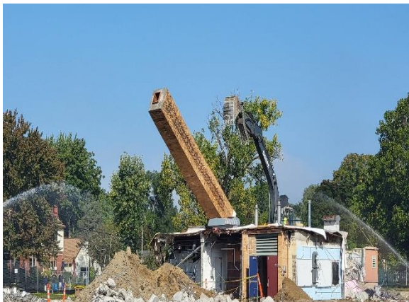
Schalm – Chimney Demolition
