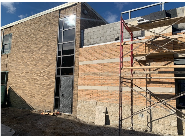
CES - Brick veneer installation
