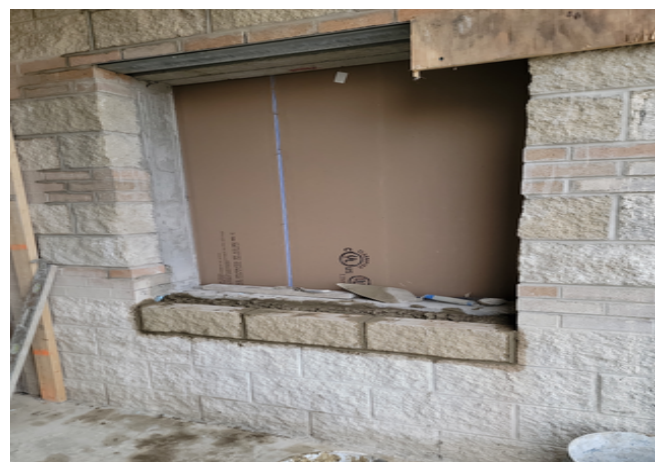
CES - Install of window sills
