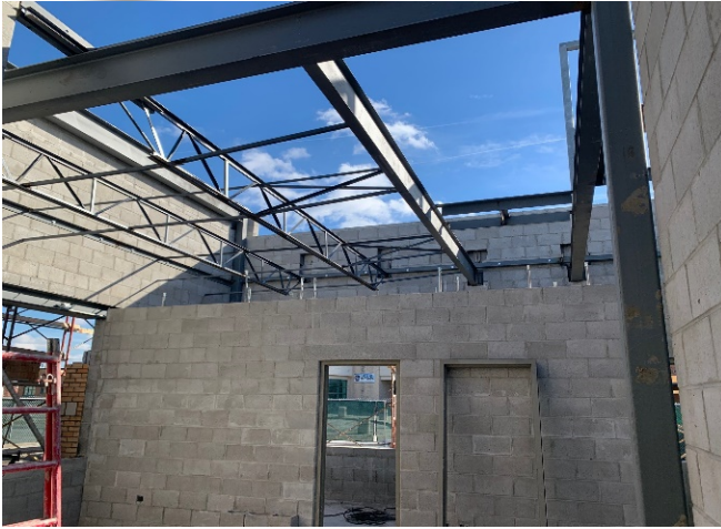
CES - Main Office Addition – Structural Steel Install
