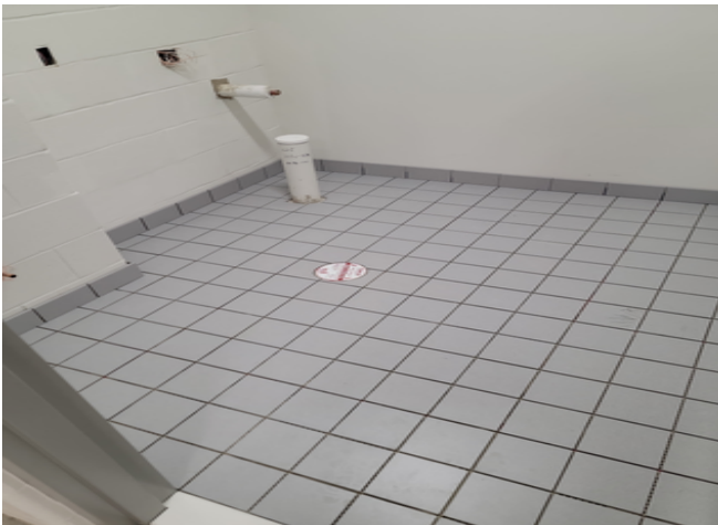
CES - Tile installation at restroom
