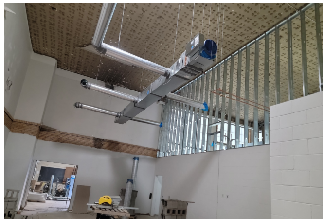
CES - interior classroom metal stub framing
