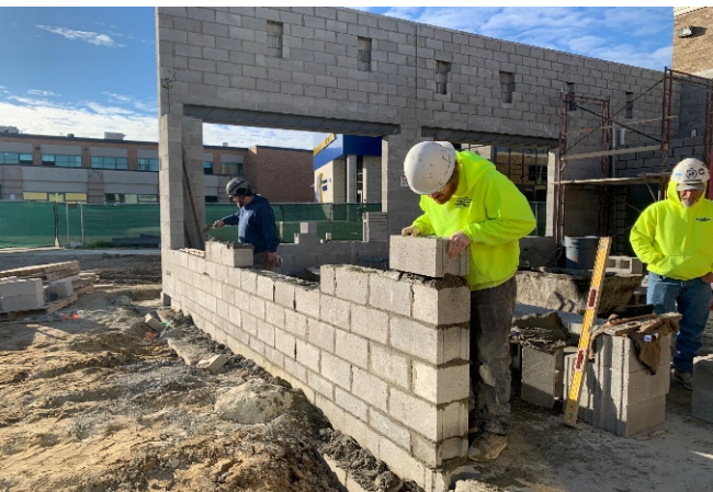
CES - front office addition masonry wall build out
