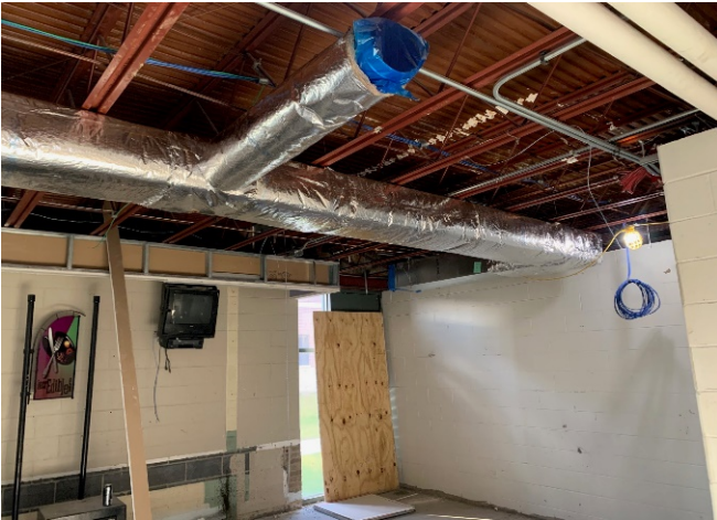
CES - HVAC duct insulation
