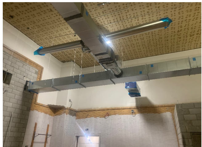
CES - mechanical duct installation
