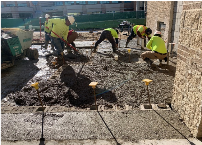
CES - slab on grade at front office addition
