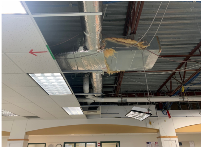
CES - ceiling and mechanical demo at Media Center
