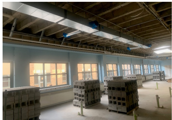
CES – mechanical duct installation
