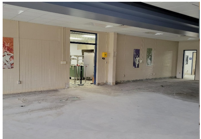
CES - cafeteria flooring demolition
