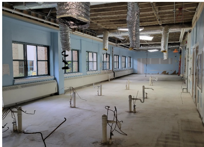
CES - classroom demolition
