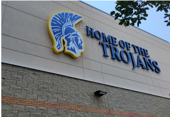
CHS - gym new sign install
