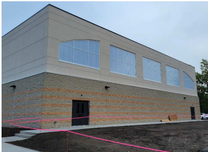
CHS - gym ready for landscaping
