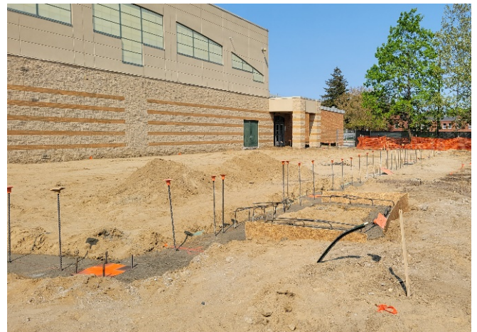
CHS – foundation concrete
