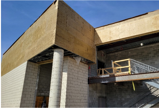
Plywood installed for metal panel locations
