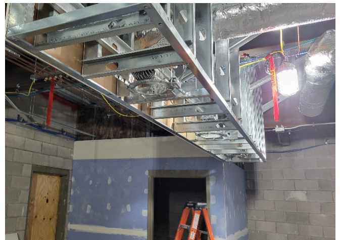
Main office soffit can lights installed
