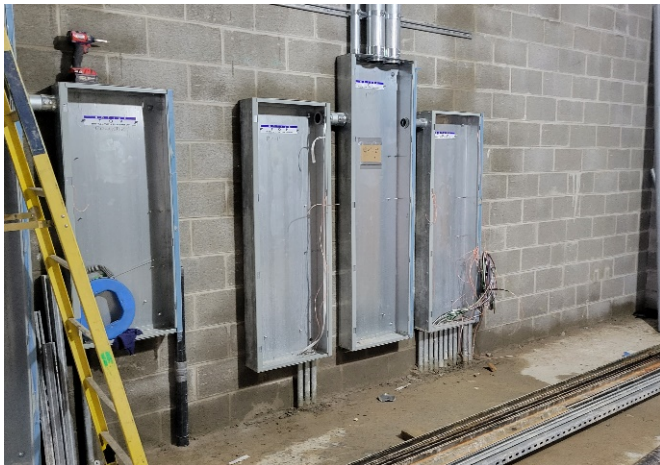
Mechanical room – electrical rough in
