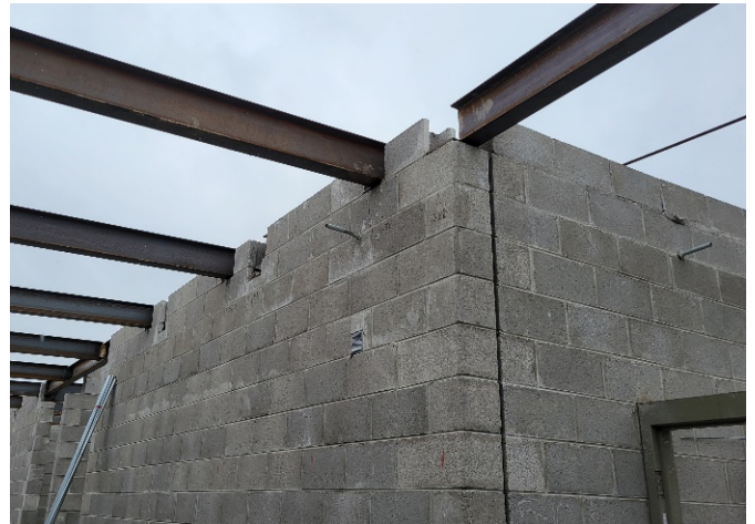
Second floor roof steel
